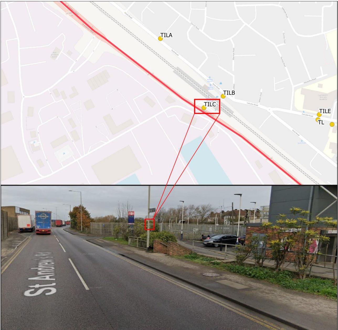
Site located in close proximity to station taxi rank and HGV parking bay serving nearby industrial areas.
